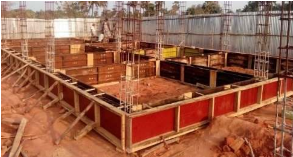
Fig.4: Plinth beam shuttering is completed
