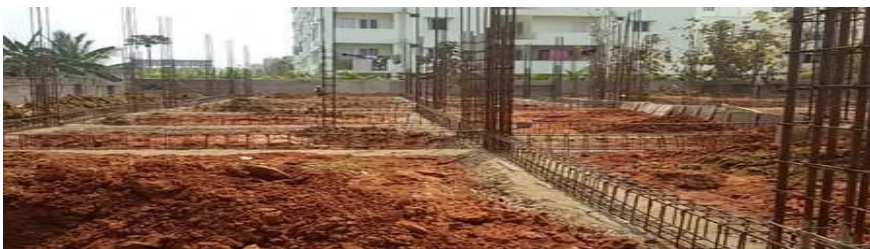
Fig.5: Reinforcement installation for plinth beams are completed
