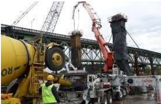
Concreting of RCC Column using Pump
