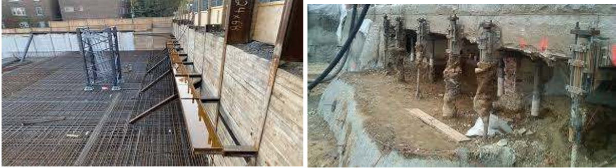
Fig. shoring and underpinning.
