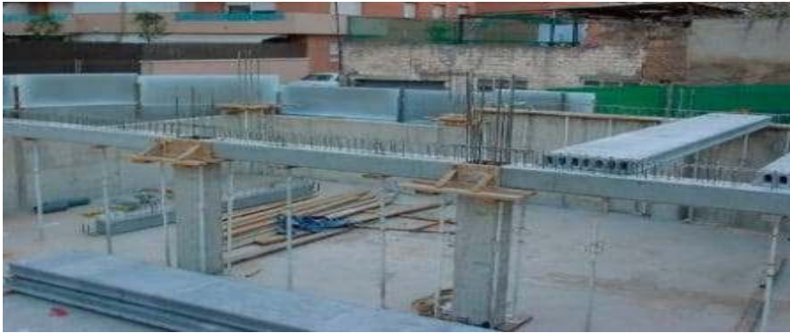
Fig. 5: Reinforced concrete beam
